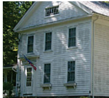
Figure 5 Mildew on Exterior
